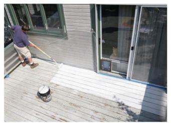
COAT THE ENTIRE LENGTH OF THE BOARDS Start at one end of a few boards and apply the entire length of the boards, to maintain a uniform texture. Clean the gaps as you go with a stir stick or a 5-in-1 style paint tool.
