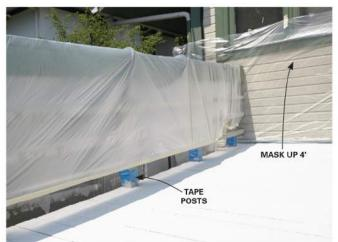
PROTECT THE HOUSE AND RAILS To avoid splattering the post rails, wrap them with masking tape and apply poly sheeting to the rails and siding. Spread poly sheeting under the deck to catch the product that oozes between the board gaps.
